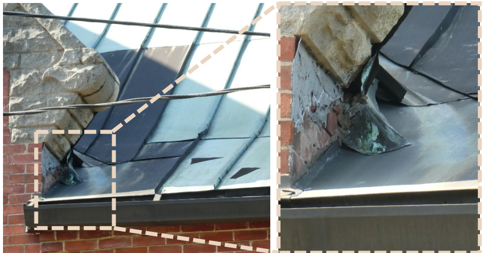
Figure 82. Previously patched area at standing seam roof. Note detached flashing at parapet wall.
