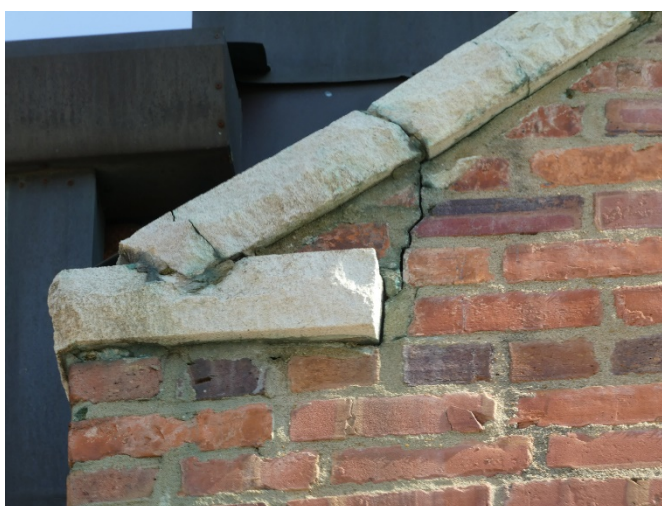
Figure 40. Cracked brick masonry and stone masonry.
