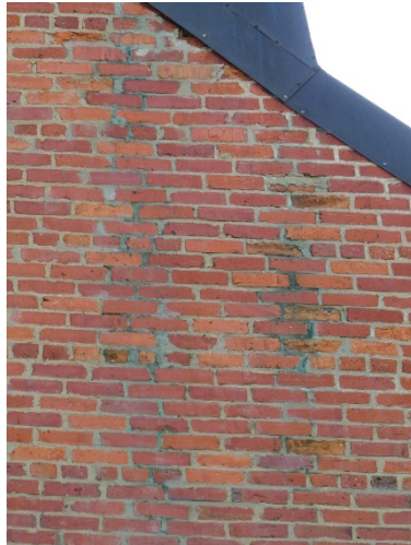
Figure 54. Biological growth at exterior walls.
