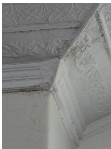
Figure 92. Water damage at interior sanctuary ceiling.
