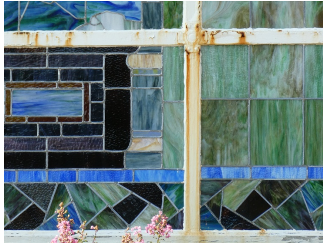
Figure 63. Minor corrosion at stained glass steel framing.
