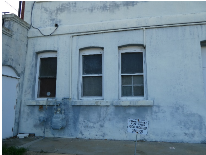
Figure 52. Water staining at exterior walls.
