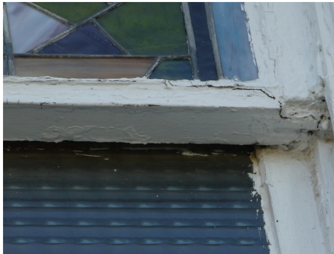
Figure 61. Cracked and split wood windows.
