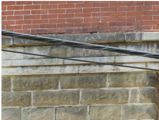
Figure 55. Biological growth at exterior walls.
