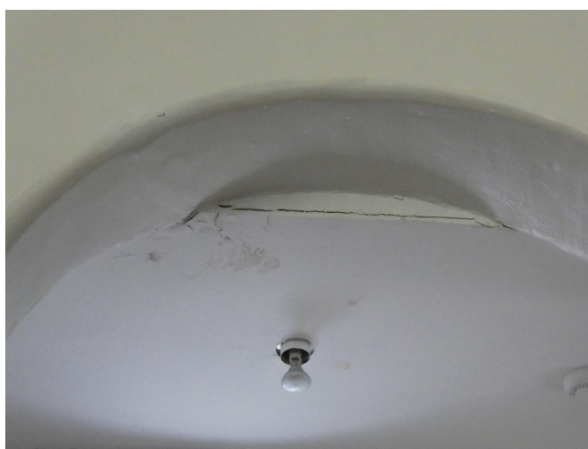
Figure 91. Water damage at interior sanctuary ceiling.
