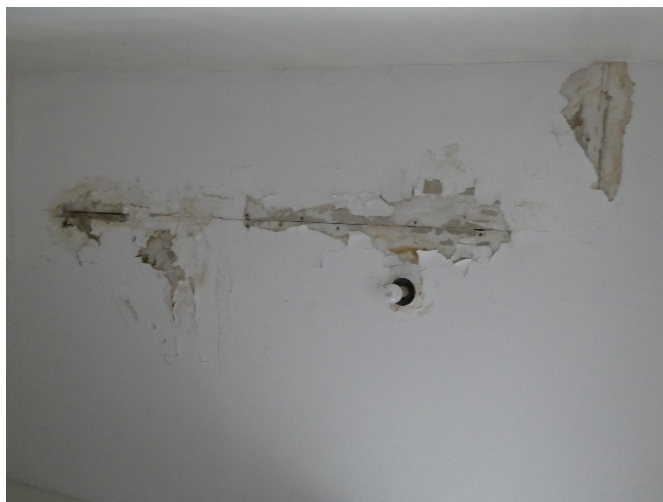
Figure 90. Water damage at interior sanctuary ceiling.
