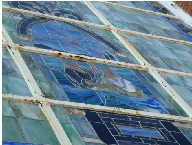
Figure 62. Minor corrosion at stained glass steel framing.
