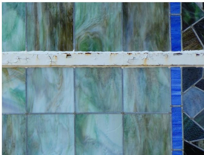
Figure 59. Peeling paint at exterior of steel-framed windows.
