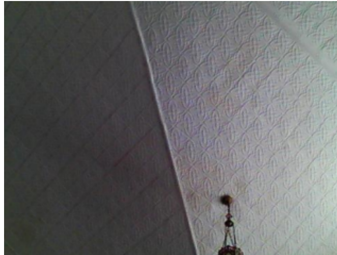
Figure 93. Interior water damage at quatrefoil tin ceiling in sanctuary.
