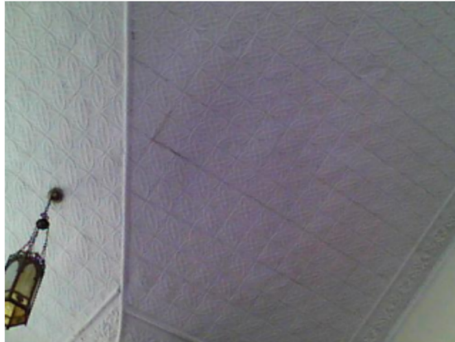
Figure 96. Interior water damage at quatrefoil tin ceiling in sanctuary.
