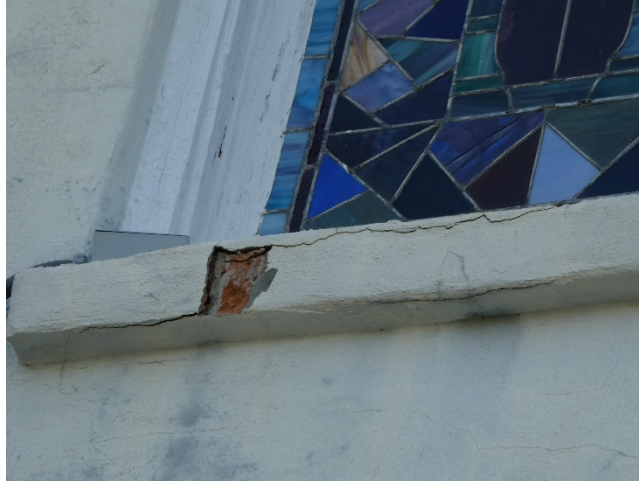
Figure 72. Cracked parge coating at window sill and spalled masonry.
