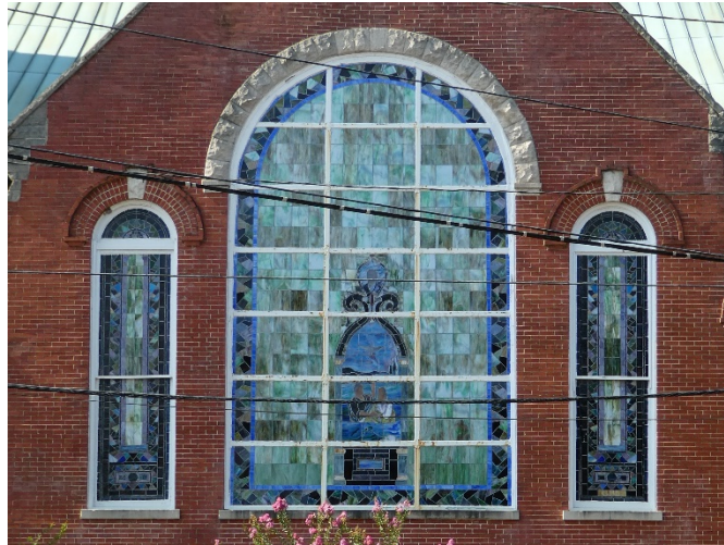
Figure 17. Stained glass windows in sanctuary. Middle window is steel framed and side windows are wood framed.
