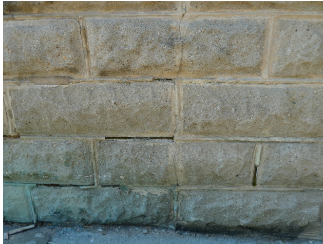
Figure 51. Deteriorated mortar joints at ashlar block.
