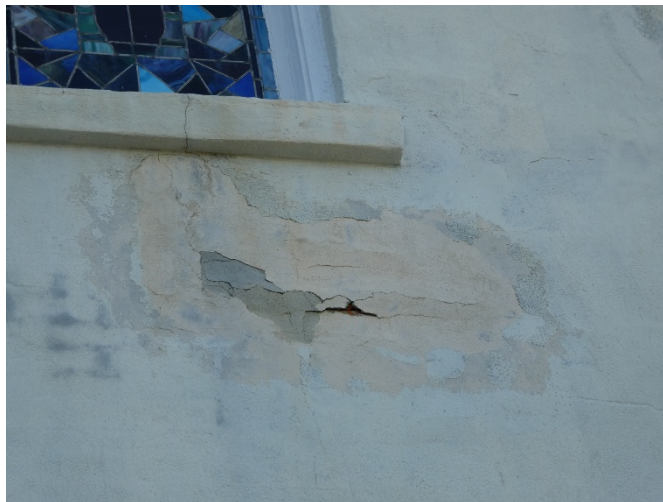
Figure 44. Cracked and spalling cement parge coating at exterior walls.
