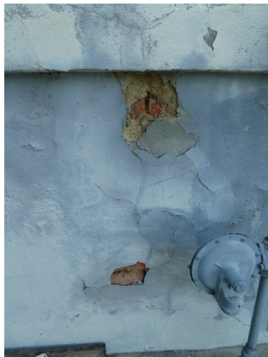
Figure 43. Cracked and spalling cement parge coating at exterior walls and deterioration of the masonry beneath.
