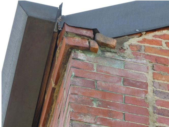
Figure 36. Displaced and loose brick units.
