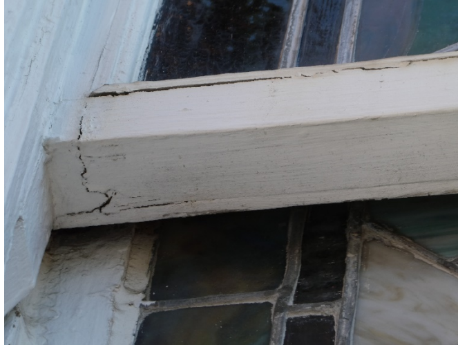
Figure 60. Cracked and split wood windows.
