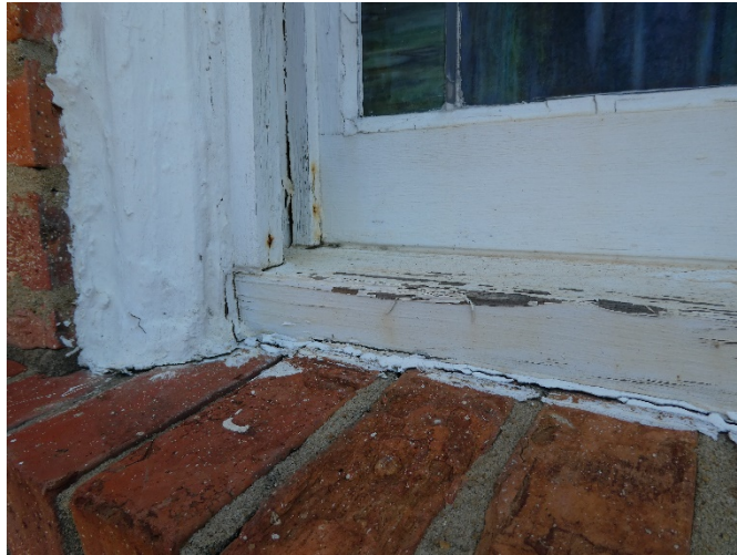
Figure 75. Deteriorated perimeter sealant.
