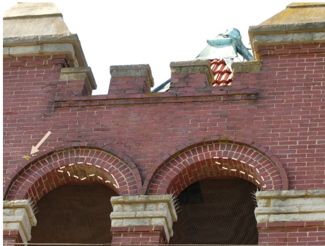
Figure 53. Efflorescence (outlined areas), biological growth (darkly stained areas) and vegetation growth (arrow) at exterior walls.
