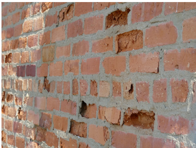
Figure 39. Eroded and spalling brick masonry.
