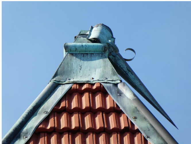
Figure 76. Detached copper finial at belltower.
