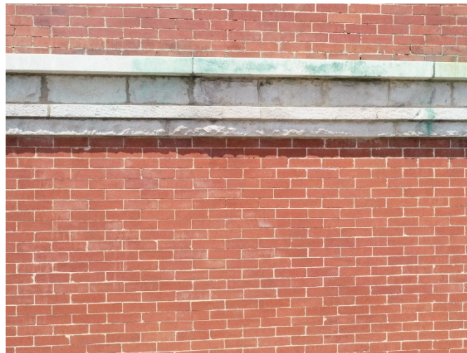
Figure 7. Typical brick masonry in running bond and stone band ornamentation.
