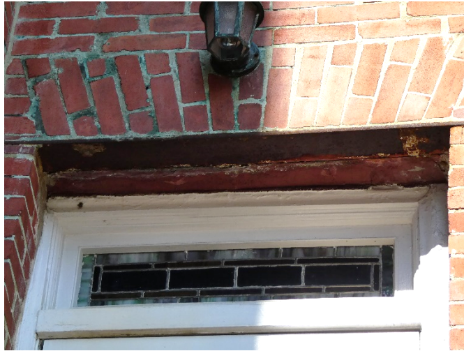
Figure 69. Minor corrosion and deflection at steel lintel.
