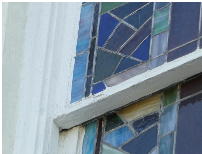
Figure 58. Peeling paint at exterior of wood-framed windows.
