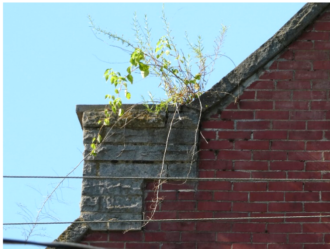
Figure 56. Vegetation growth at exterior wall and roof copings.
