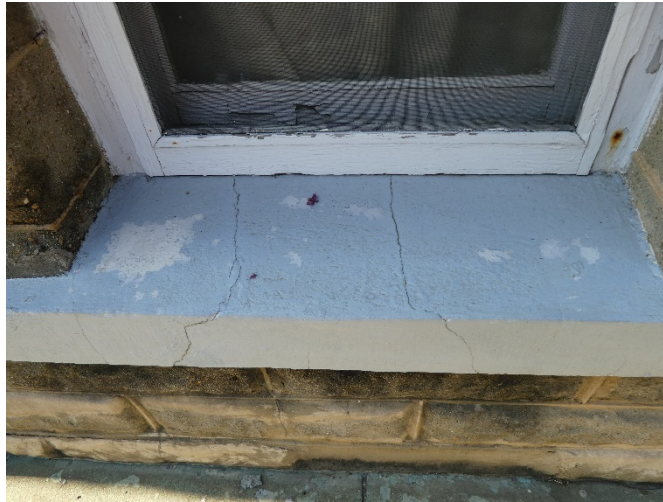
Figure 73. Cracked parge coating at window sill.
