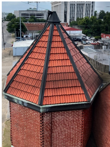
Figure 77. Detached copper finial at southeast tower.
