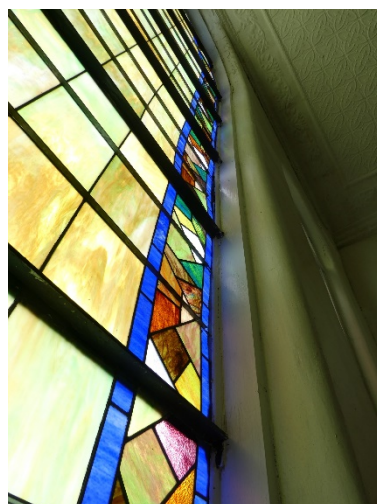
Figure 65. Areas of deflection at steel-framed stained glass windows.
