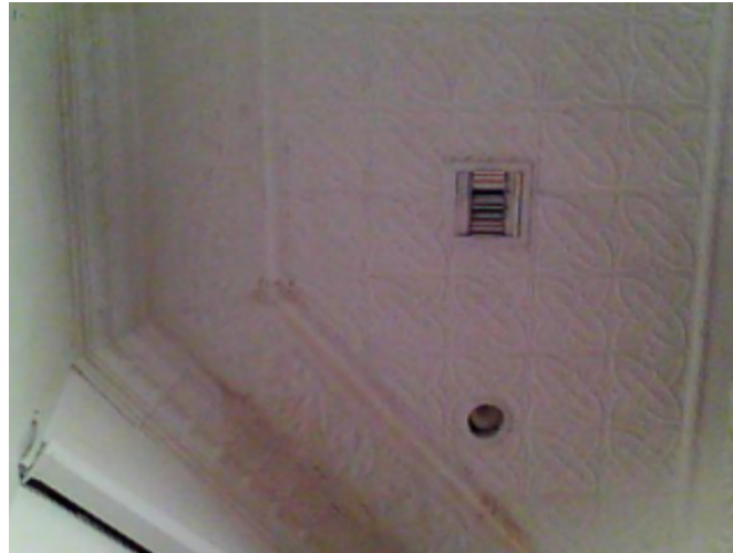
Figure 99. Interior water damage at quatrefoil tin ceiling in sanctuary.
