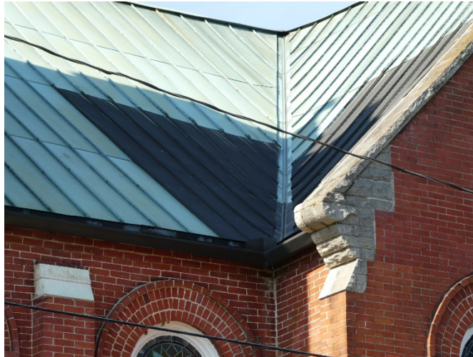
Figure 81. Previously patched areas at standing seam roof (black areas).
