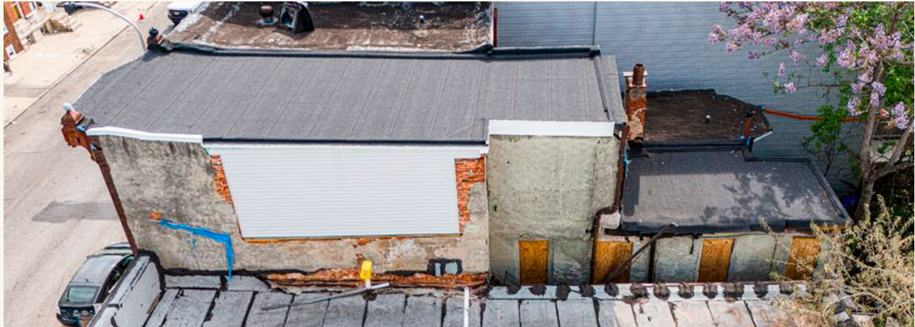
Fig. 4. The H.O. Tanner House, view of the west (side) elevation. The 1 ½ story wing of the Mt. Lebanon Baptist Church is in the foreground. Atmos Imagery, 2024.
